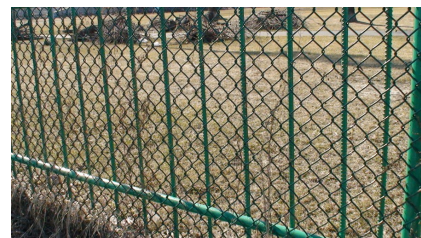
Initially a chain link fence, this fence required modification to prevent persons from simply cutting the fabric. Both an example of good risk management and infrastructure management, but also an example of issues that can lead to rework
